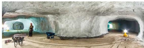
*Figure 1: With the ground supporting shotcrete in place, the CASPAR cavern on the 4850 Level is ready for outfitting*
