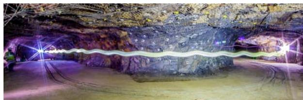
*Figure 5: Shotcrete will soon cover these rock walls to make the area safe for the CASPAR experiment. (SURF Photographer Matt Kapust used battery-powered LED light to illuminate the cavern over a long exposure.)*
