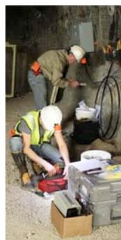
*Figure 3: Jamey Tollefson, Industrial Technician, and Tanner Prestegard, University of Minnesota grad student, connect fiber optics for the seismometers on the 4850 Level*
