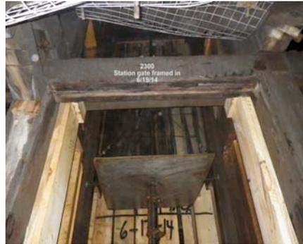
Figure 6: Framed-in new support for Station Gate at 2300 level
