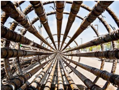
Figure 4: Rebar is tied together as a long cylinder
